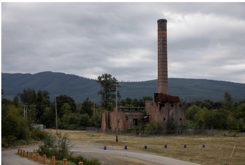
An old sawmill seen in Snoqualmie, a small but growing town in eastern King County, Washington. The city wants to turn the area into apartments, wine bars, restaurants and offices. But first the city, state and county have to figure out if the project is safe and doable. (Matt M. McKnight/Crosscut)
